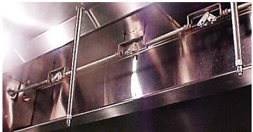
Fire-extinguishing system distribution nozzles and detection links. Note required grease caps are missing from the appliance nozzles.
