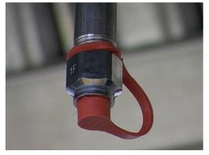
UL 300 1 flow Ansul nozzle with rubber-type blow-off cap
