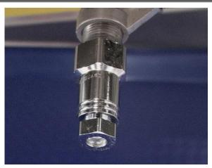
Range Guard/Kidde UL 300 appliance nozzle. Note: Aluminum grease seal at base of nozzle
