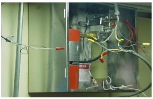
Improperly wired extinguishing system control components. Installation and service should only be performed by properly trained individuals. Note: This is a red-tank Ansul and no longer factory compliant.
