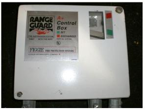
Range Guard A+ mechanical control head
